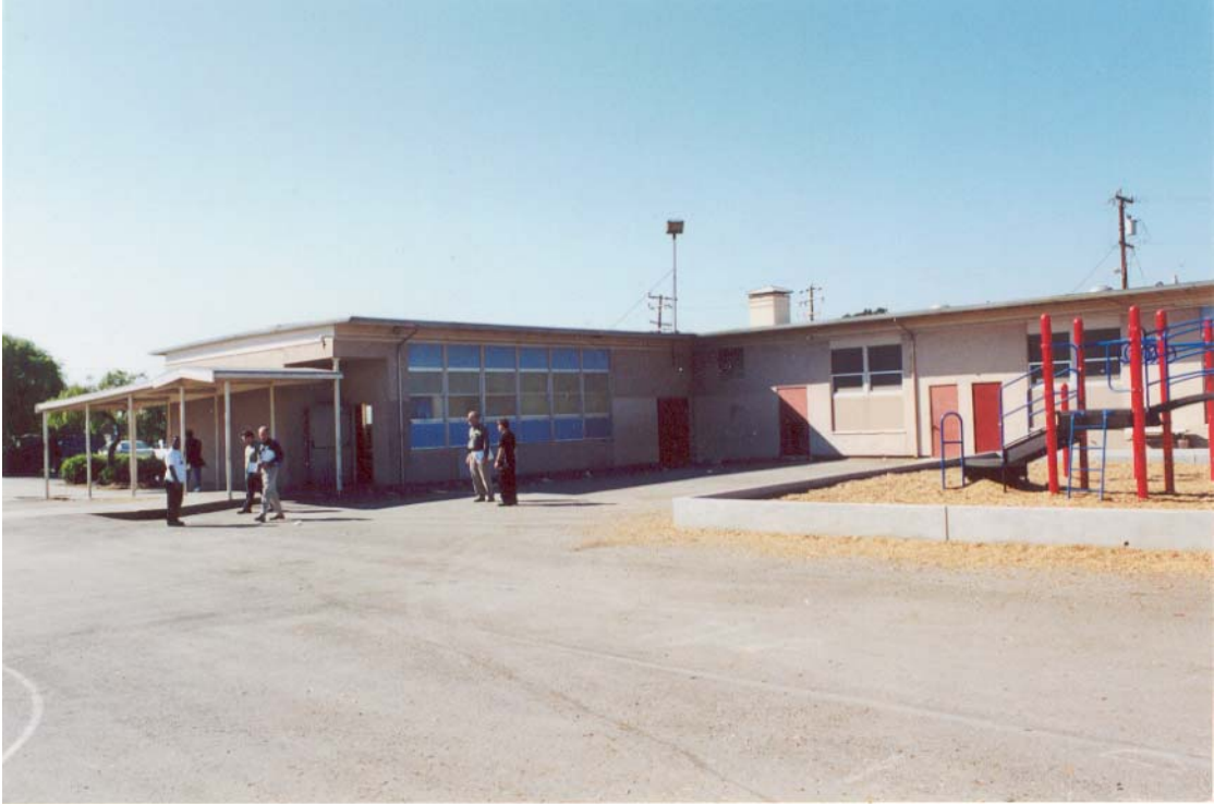
Figure 8: 1944 Classroom and Covered Walkway
